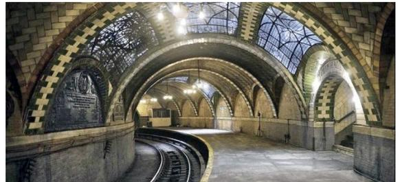
The original City Hall station, designed by architects Heins and LaFarge. With an arched, tiled ceiling constructed by Rafael Guastavino, this station was the showpiece of the subway system. Skylights and chandeliers with the newest electric lights illuminated the now-abandoned station.
